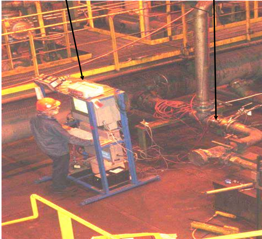
Figure 4. Instrumentation and probe installations in the field.
